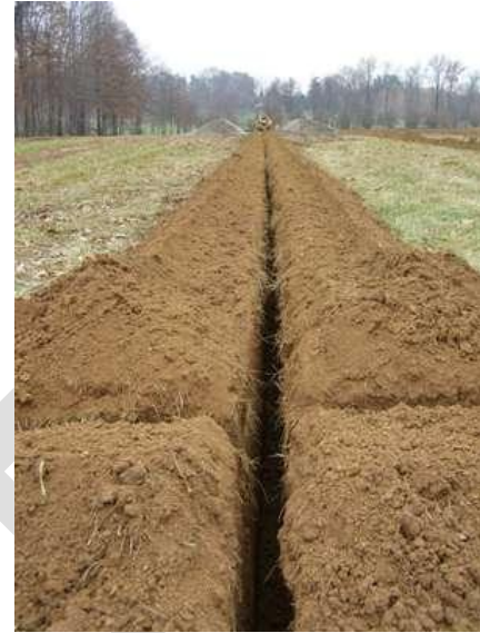
4" drain tile ditch with a layer of river rock
