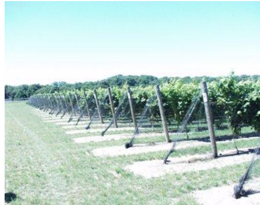
Wood end assemblies on Long Island
