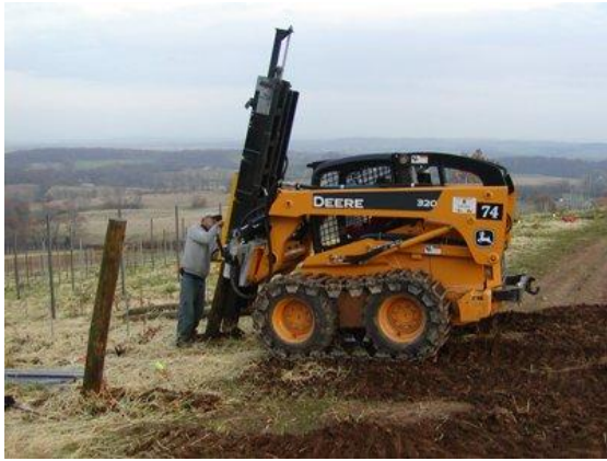
Proper equipment and method to install end posts
